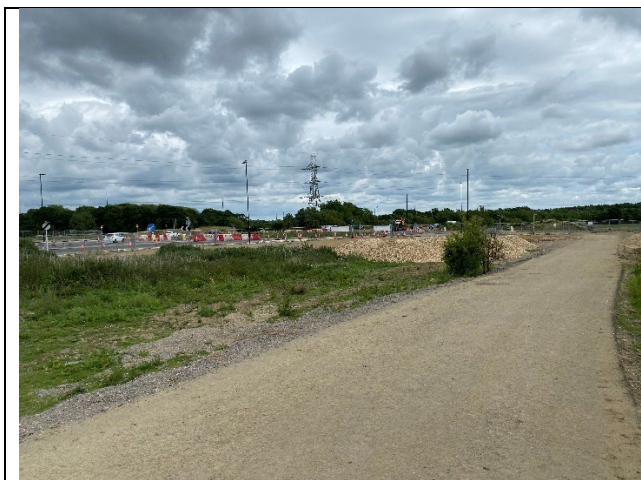
Western Link Road under construction
