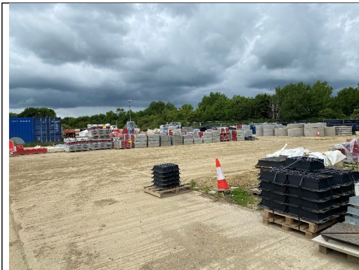
Existing temporary highways compound
