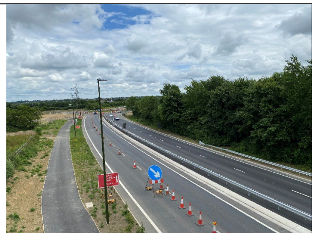
Newly widened A2300 past the site
